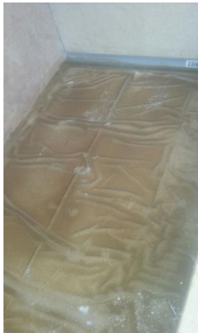
Figure 2: Wrinkles occurred when the molded part was left in the garage.
